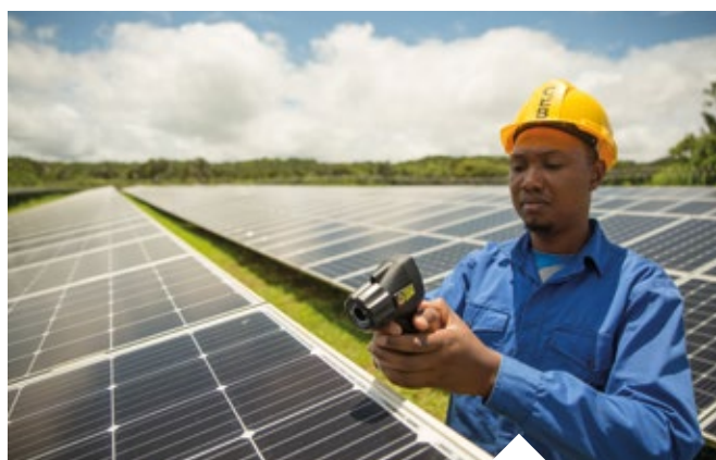
The photovoltaic farm covers an area of 20,000 m 2 and comprises 5,900 panels, Henrietta, Mauritius.
